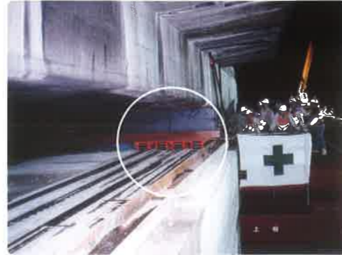
橋梁撤去工事 (NEWS 0192) Removal work of a bridge girder
