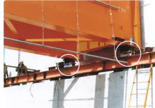
橋梁工事 (NEWS 0125) Bridge girder construction
