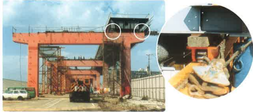
橋梁横取り工法 (NEWS 0150) Side-tugging method of bridge girder
